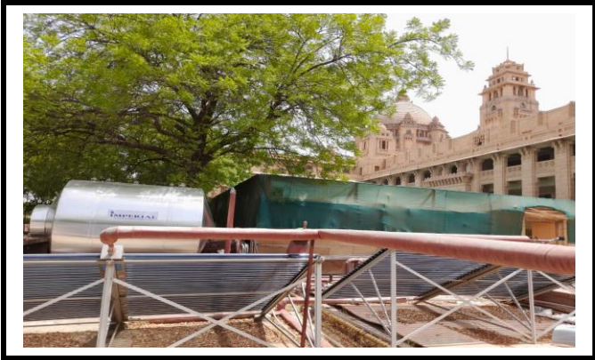
5000 LTR FULLY AUTOMATED SOLAR WATER HEATER, UMAID BHAWAN, JODHPUR, RAJASTHAN
