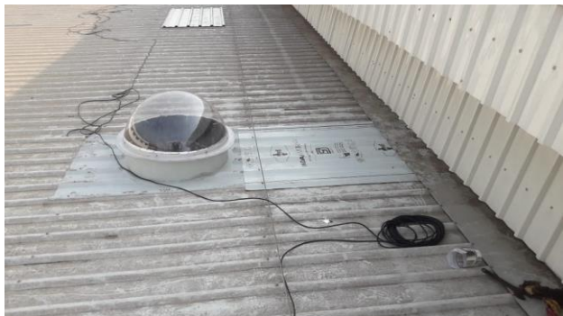
400 WATT EQUIVALENT SOLAR DAY TUBE, FLENDER DRIVES PVT. LTD.
