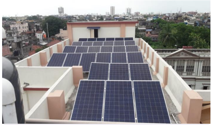
10KW ON-GRID SOLAR POWER PLANT, RAMMOHAN COLLEGE, KOLKATA,
