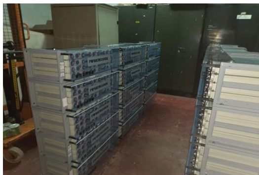
SOLAR BATTERY BANK – 360V 100AH CENTRE FOR DEVELOPMENT OF ADVANCED COMPUTING , THIRUVANANTHAPURAM, KERALA
