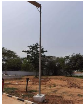
30 WATT HYBRID SOLAR STREET LIGHT, VANIKI MAHAVIDHYALAYA, MUNGER
