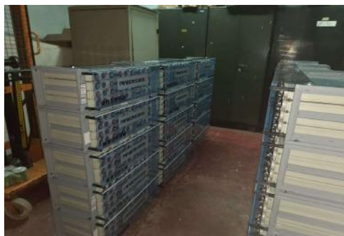
SOLAR BATTERY BANK – 360V 100AH CENTRE FOR DEVELOPMENT OF ADVANCED COMPUTING , THIRUVANANTHAPURAM, KERALA
