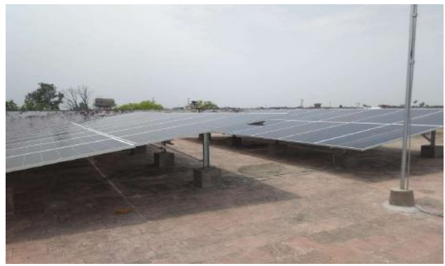
40 KWP ON-GRID SOLAR POWER PLANT CIVIL COURT NAWADA, BIHAR
